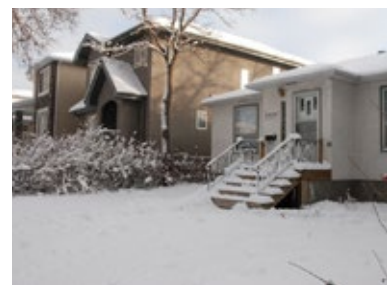
Density is beginning to increase in some mature neighbourhoods.
