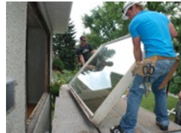
Increasing the energy efficiency of a residential building by replacing windows.
